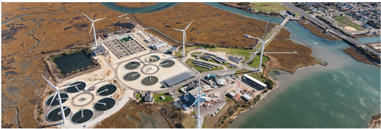
Aerial view of Atlantic County Utility Authority. Photo credit: ACUA
